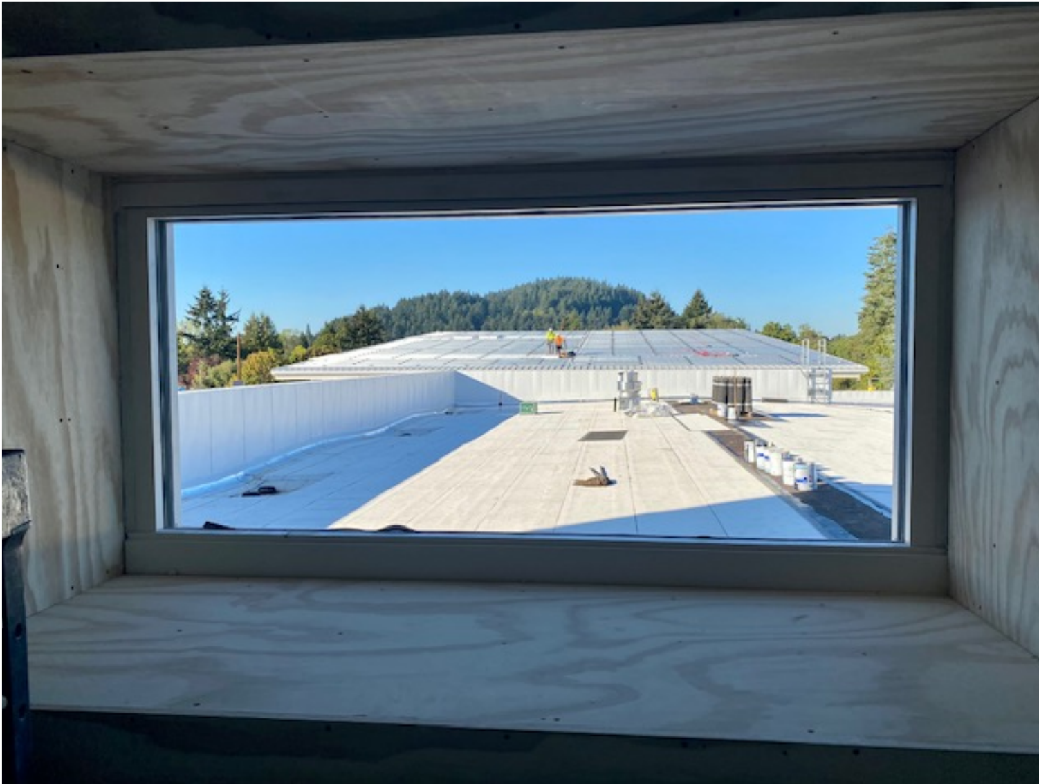
View of Roof & Solar PV Array / October, 2020
