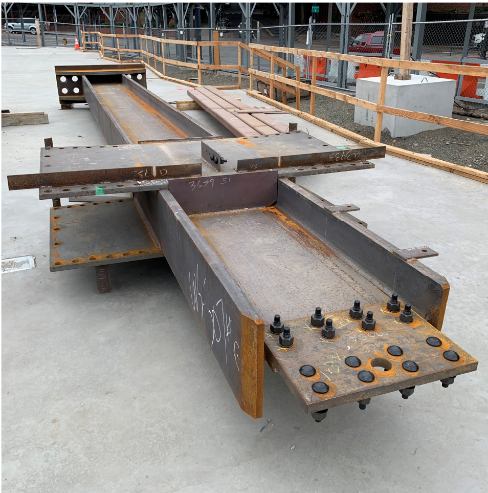
Steel column with Sideplate connection.
